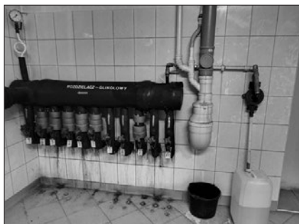
Fig. 3. Glycol manifold in the VGHE installation – glycol return to the building
