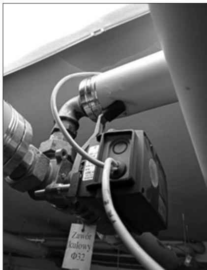
Fig. 4. The regulating element of the three-way valve immobilized by heating pipe insulation
