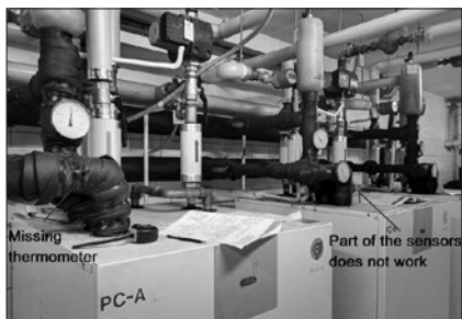
Fig. 5. Missing or malfunctioning thermometers and manometers
