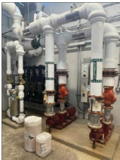
Fig. 7. Cascade of air-source heat pumps in the Primary School in Dęba, Poland [84] (on the left) and installation of a ground-source heat pump – supply and return from the ground heat exchanger in Buckley Elementary in Connecticut, USA [85] (on the right)
