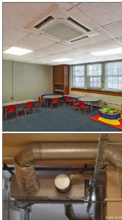
Fig. 6. Examples of ventilation and air conditioning systems' units in school buildings: VRF cassette indoor unit [79] (on the left) and heat recovery unit (recuperator) [80] (on the right)
